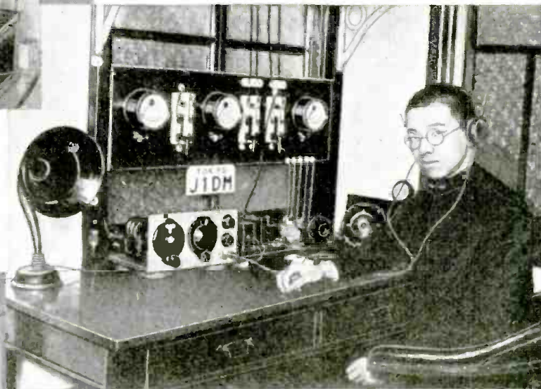
Shades of Heinrich Hertz! Yep—a Ham station of 1916 vintage! Transmitter, receiver, an' everything. On the wall is a membership certificate of the "Radio League of America," established by Hugo Gernsback, editor of this magazine. This station operated on 200 meters, real short for that period, and the receiver was a "1-tuber," observable in the center of the photo. Note the rotary spark gap at the right and the oscillation transformer made of copper ribbon, just below the gap! Roswell J. Parker.
